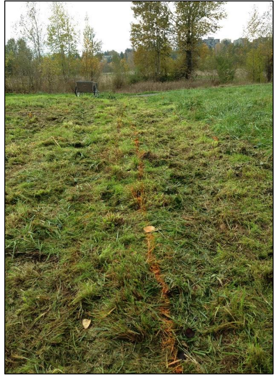
Picture 2: Glo-paint was used to mark the center of the trench. Volunteers started at the center line and dug outward.
