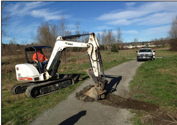
Picture 11 (Above) and 12 (Right): The UW Heavy Machinery team helped to install the pipe under the trail using a bobcat and a dump truck.
